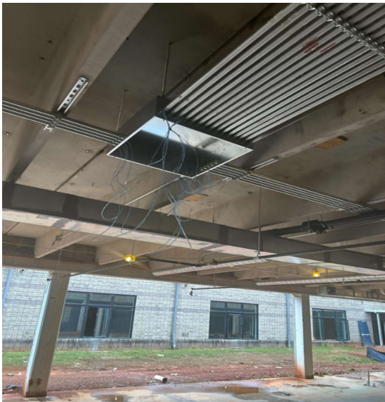
Continue installing conduit and raceway boxes throughout
