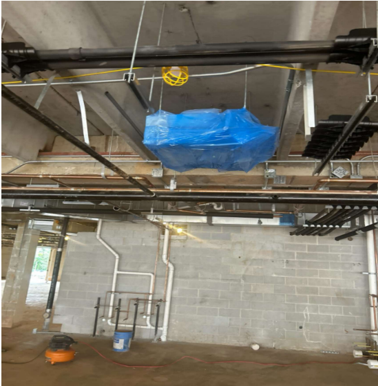
Continue Installing branch selectors in area 3 level 1
