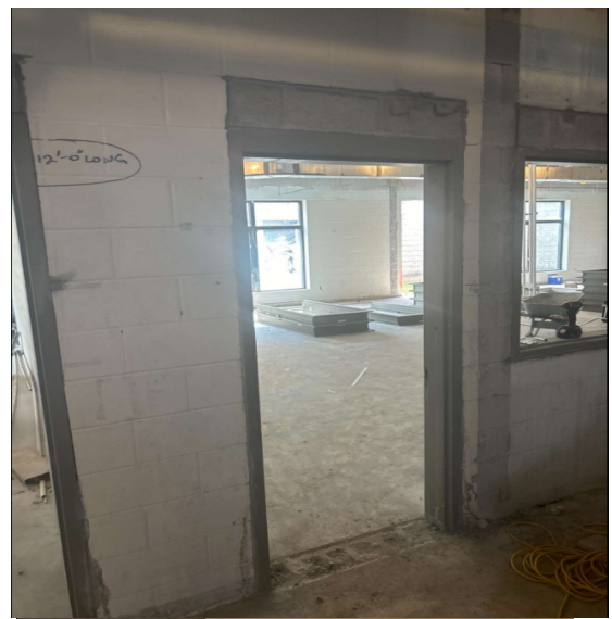
Continue installing hollow metal frames in area 2
