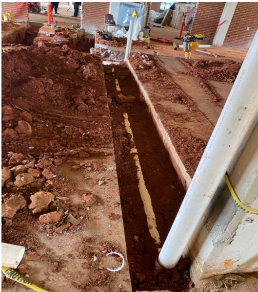
Continue underground plumbing backfill in corridor area 3
